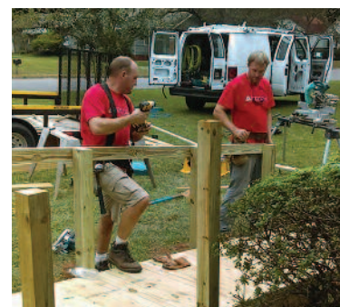
A crew from the Church of the Highlands installs a new ramp at the Downings’ home.
